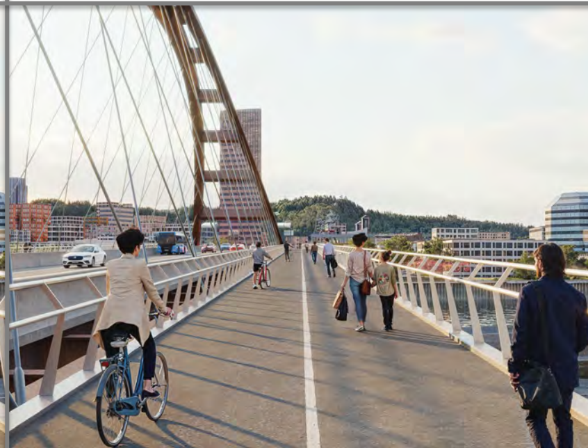
Braced basket-handle arch
