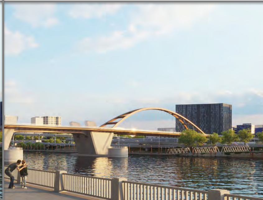
Braced basket-handle arch
