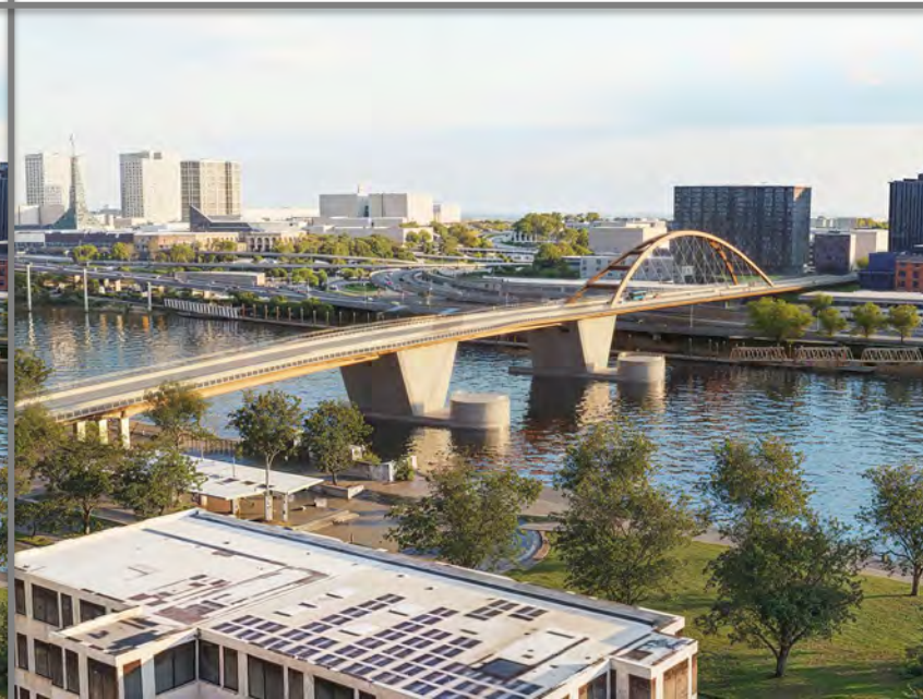
Braced basket-handle arch
