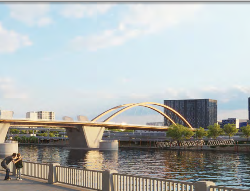
Unbraced through arch
