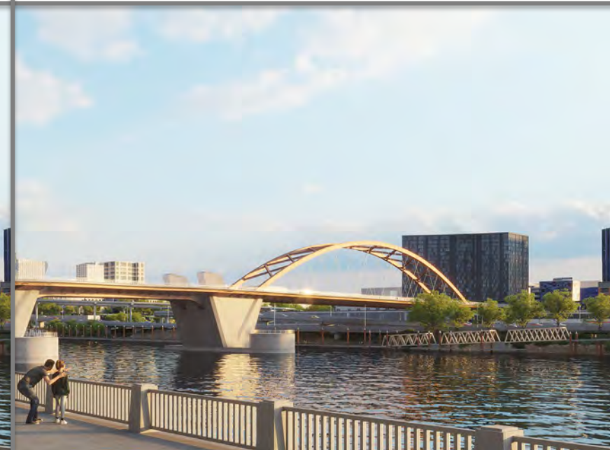
Braced vertical arches
