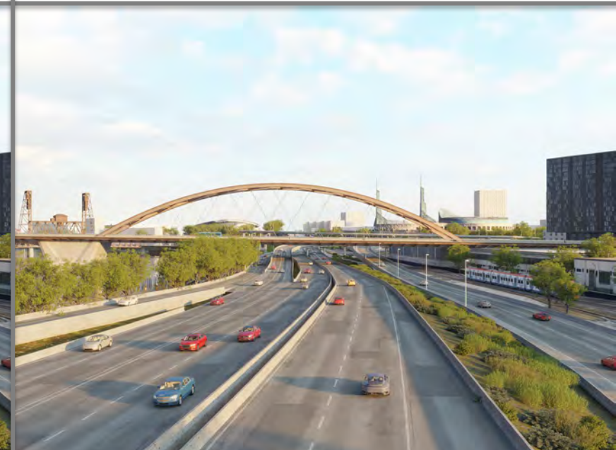
Braced vertical arches
