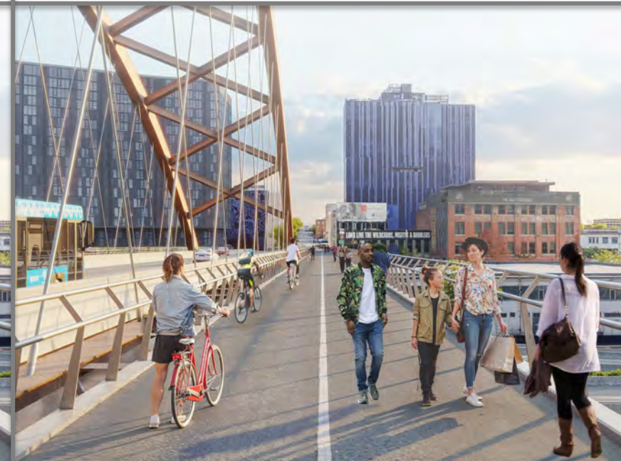
Braced vertical arches
