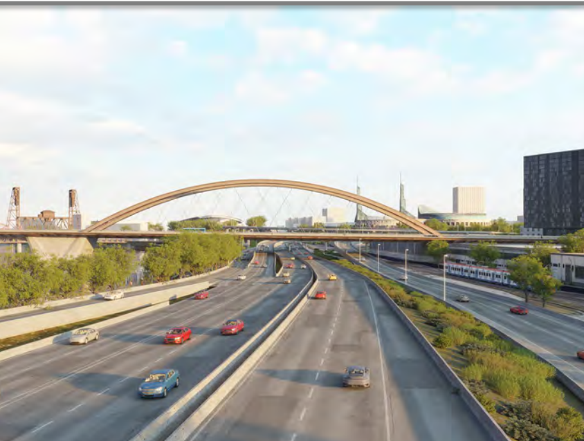
Unbraced through arch
