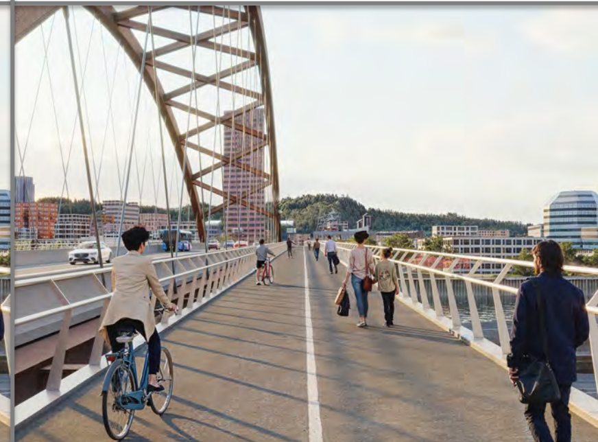
Braced vertical arches
