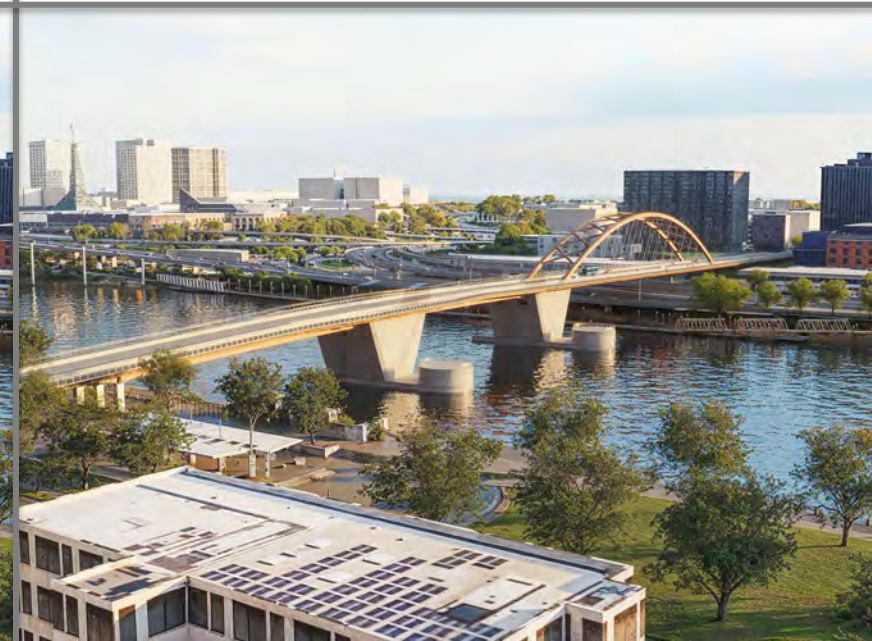
Braced vertical arches
