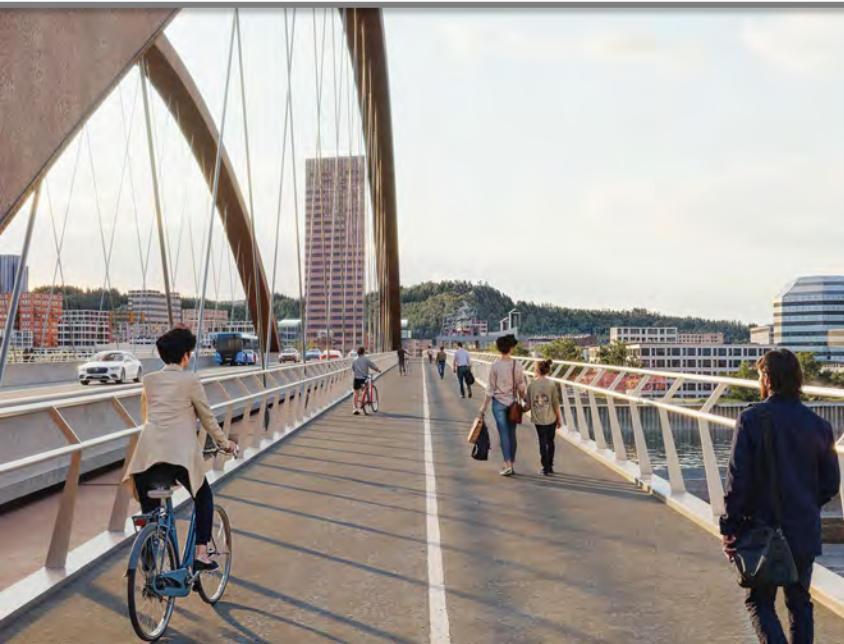
Unbraced through arch
